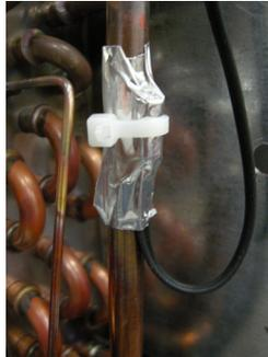
Thermistor attached to the refrigerant line.
