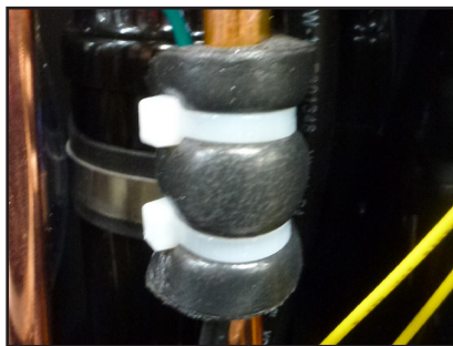
Figure 8: Thermistor attached to the refrigerant line.
